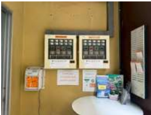
Fire Alarm Control Panel
